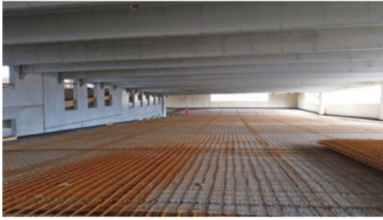
Typical Topping Slab Preparation. Mesh Installed, Edge Felt Installed.
