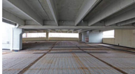
Slab Preparation, Level 2 – Rain Water Leaders Installed, Joints Prepared for Topping Slab.
