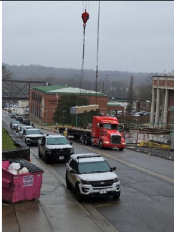
Setting Column in Southwest Corner of Structure
