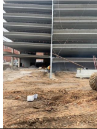
Progress of Precast Erection on 2/9/24
