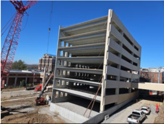
Progress of Precast Erection on 2/5/24
