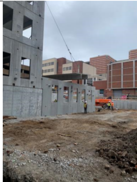
Light Wall Installed, Setting Double Tee Along Drive Ramp
