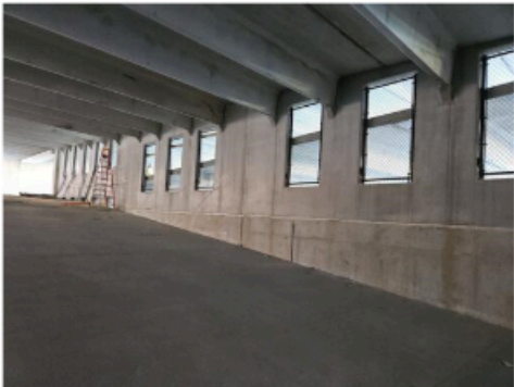
Installation of Fence Inserts at Litewall
