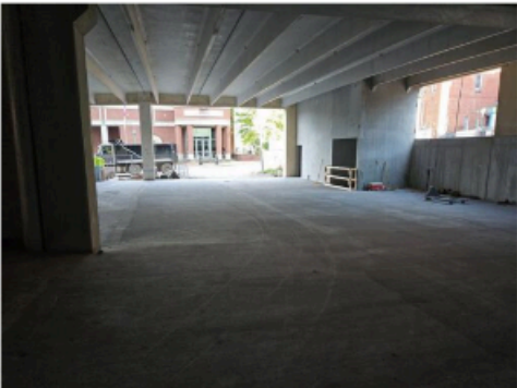
Level 0 Concrete Completed
