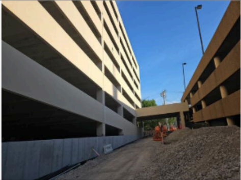
Preliminary Grading and Underground Utility Work at Cumberland Alley
