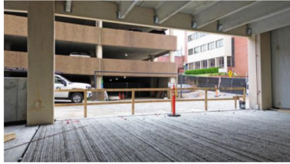
Secured Entrance to CC1SPG at Commerce.
