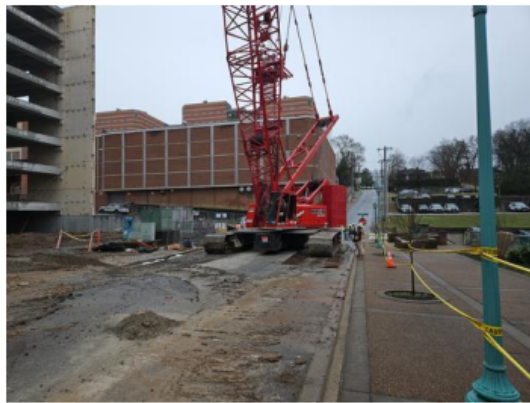
Crane Positioning for Final Sequencing.
