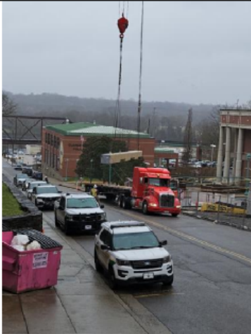
Setting Column in Southwest Corner of Structure
