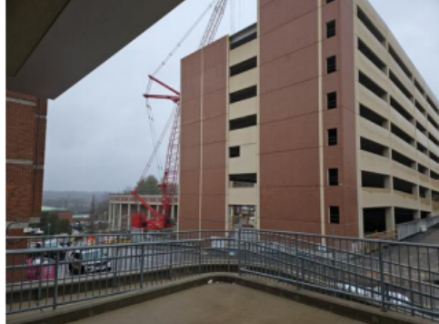
View of South Elevation. Completing Last Bays of Erection in Southwest
