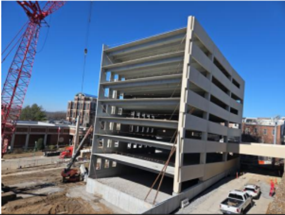
Progress of Precast Erection on 2/5/24
